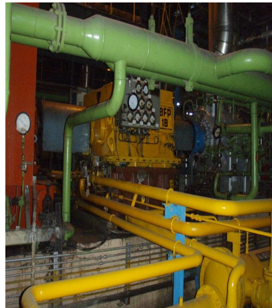
Figure 5: Boiler feed water pump
