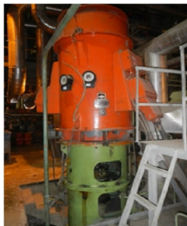
Figure 9: Condensate Extraction Pump
